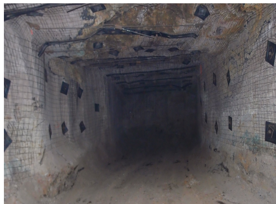
Fig. 6. Control of mine tunnel deformation by sidewall rock bolting
