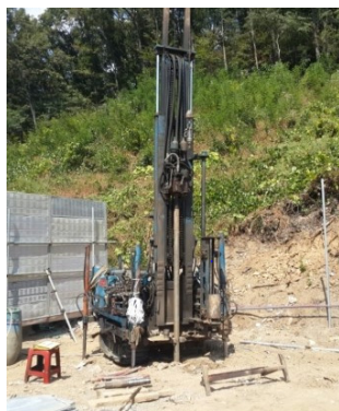
(a) In-situ boring
